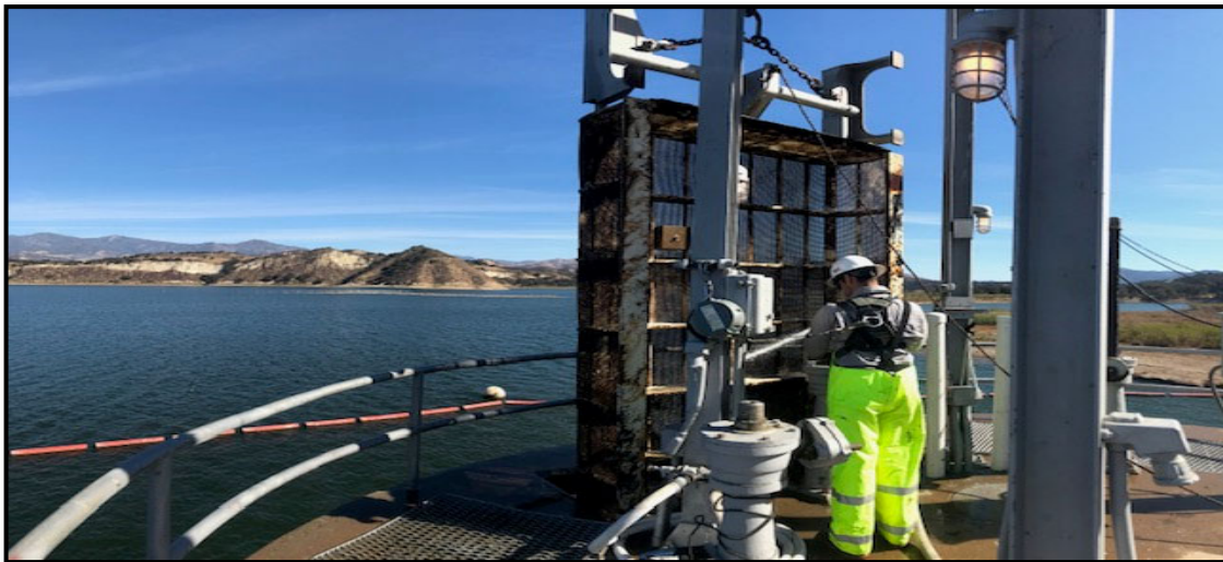
North Portal Intake Tower
