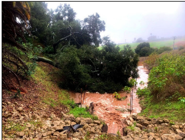
Lauro Reservoir - Main Debris Basin
