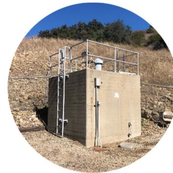
Figure - Lauro Outlet Works Tunnel Access House
