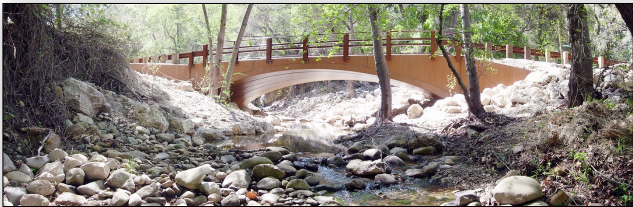
Quiota Creek Fish Passage Project
