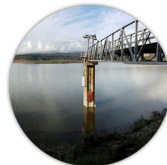
Figure - North Portal Intake Tower
