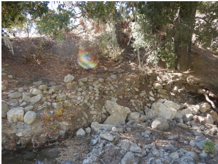
Figure 10: Quiota Creek Crossing 1 showing the post-project (As-Built) condition.
