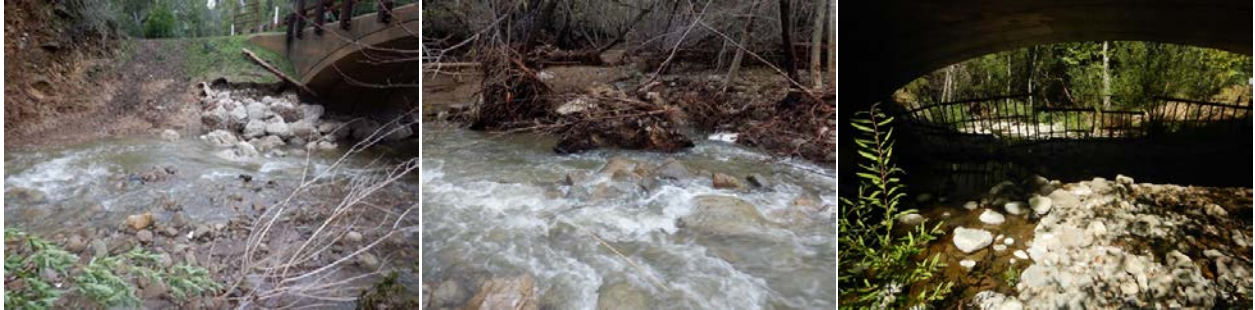
Figure 7: Quiota Creek Crossing 8 showing the pre-project condition.
