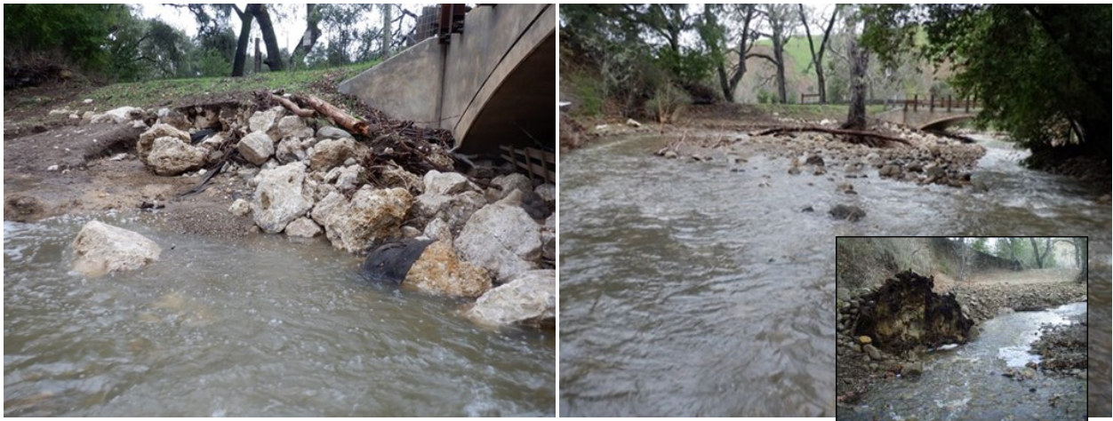
Figure 3: Quiota Creek Crossing 4 showing the pre-project condition.
