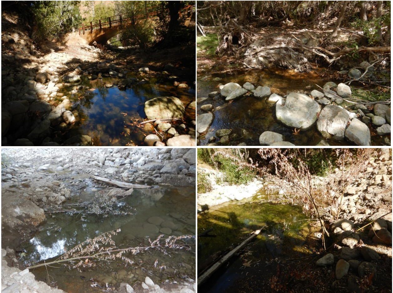
Figure 8: Quiota Creek Crossing 8 showing the post-project (As-Built) condition.
