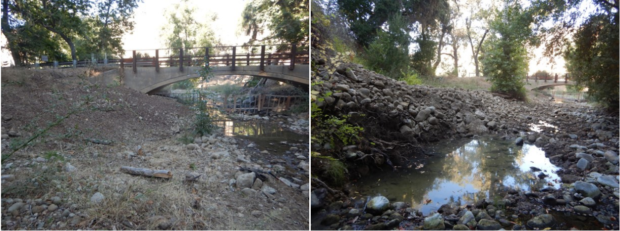
Figure 4: Quiota Creek Crossing 4 showing the post-project (As-Built) condition.
