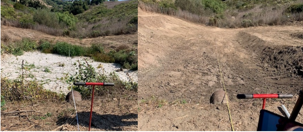
Figure 6. Boy Scout Debris Basin Sediment Removal
