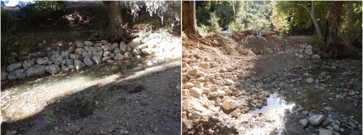
Figure 6: Quiota Creek Crossing 3 showing the post-project (As-Built) condition.
