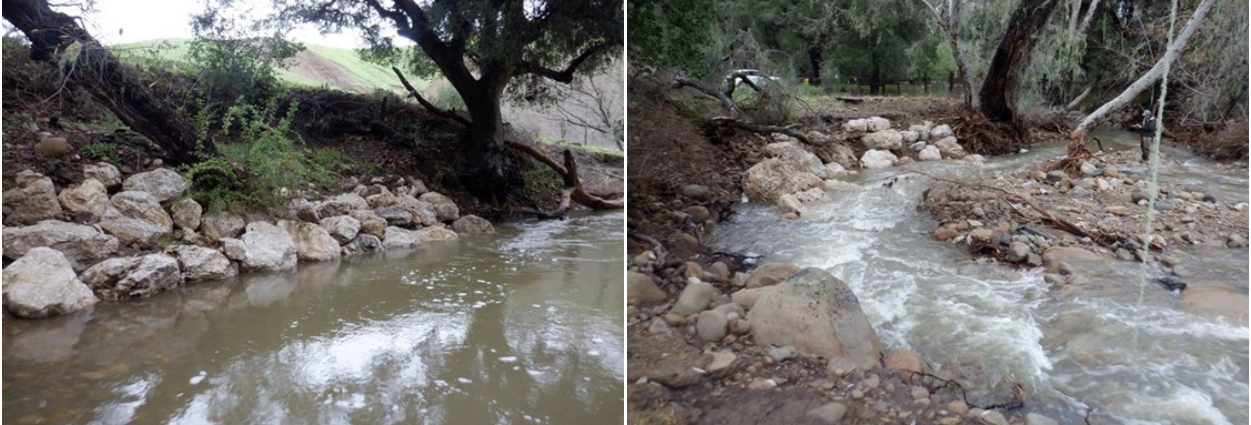
Figure 5: Quiota Creek Crossing 3 showing the pre-project condition.
