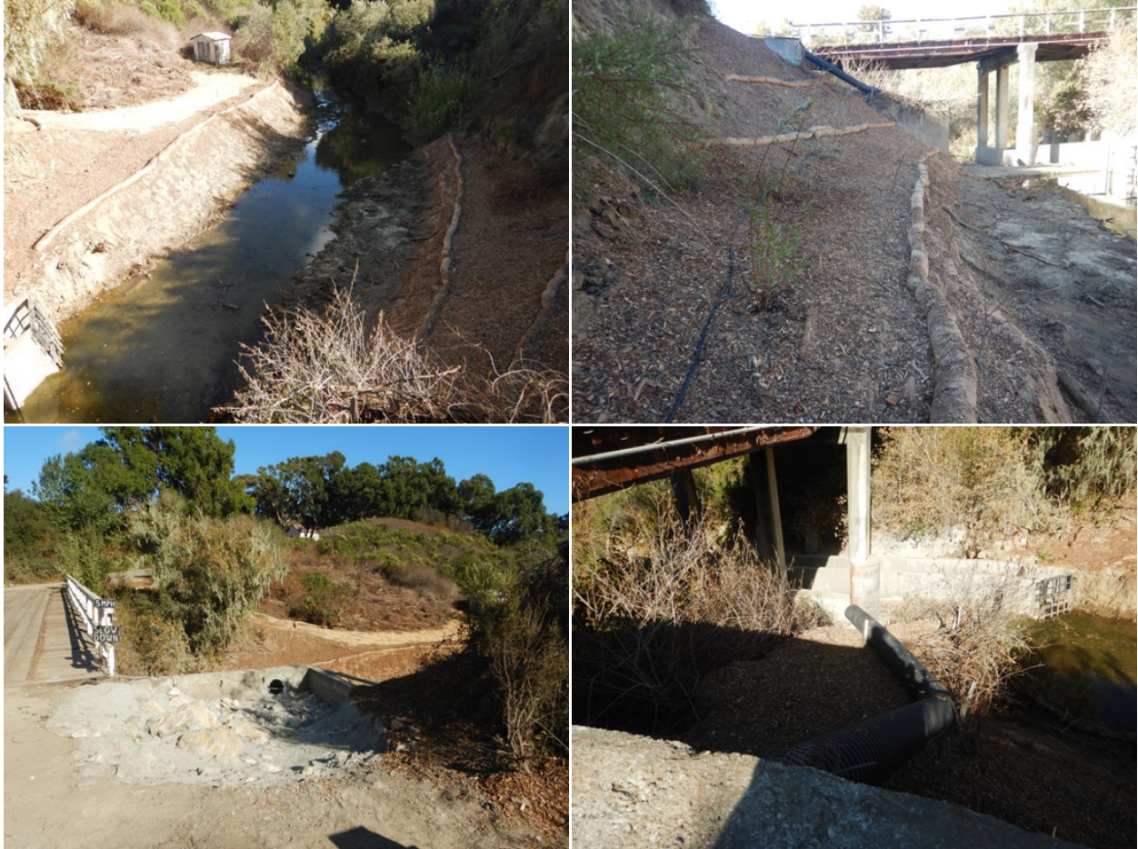
Figure 2: El Jaro Creek at Rancho San Julian fishway showing the As-Built (current) condition with the stabilized western bank, removed aggregated sediment on the eastern bank, partially straightened stream channel, road drain fix, and revegetation.
