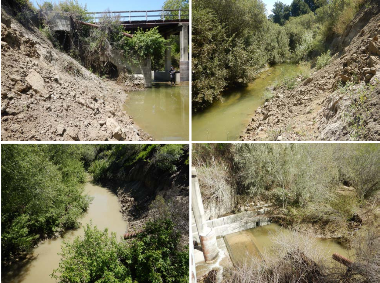
Figure 1: El Jaro Creek at Rancho San Julian fishway showing the pre-project conditions of bank failure, sediment aggregation, and partial occlusion of the upstream entrance to the fishway.
