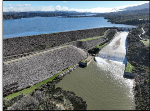
Bradbury Dam Spillway following the February 2024 storm event.
