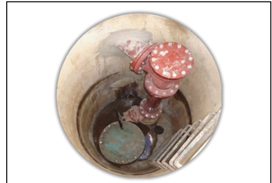
Figure - Inside of Blow Off Structure
