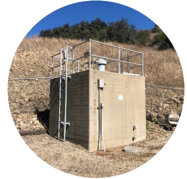
Figure - Lauro Outlet Works Tunnel Access House
