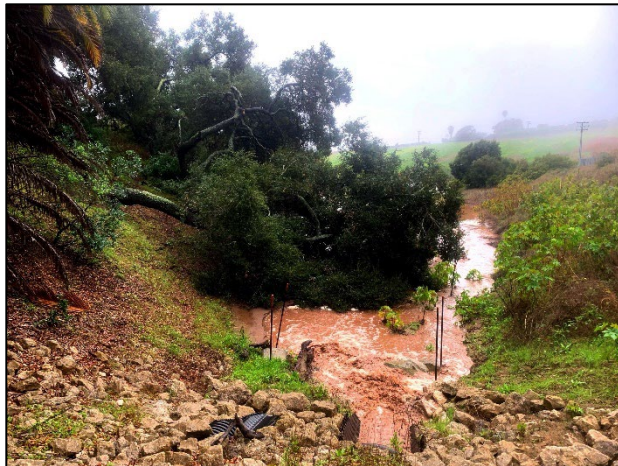
Lauro Reservoir - Main Debris Basin
