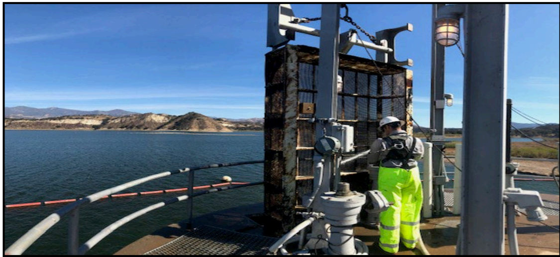
North Portal Intake Tower
