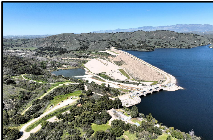
Lake Cachuma Bradbury Dam, March 2024
