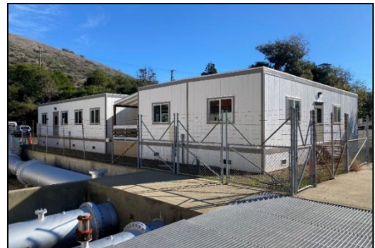
COMB Office Buildings
