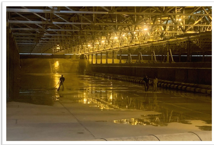
Ortega Reservoir Maintenance Project
