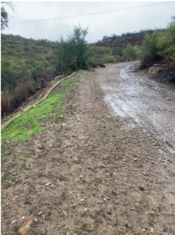
North portal access road slide repair and drainage
