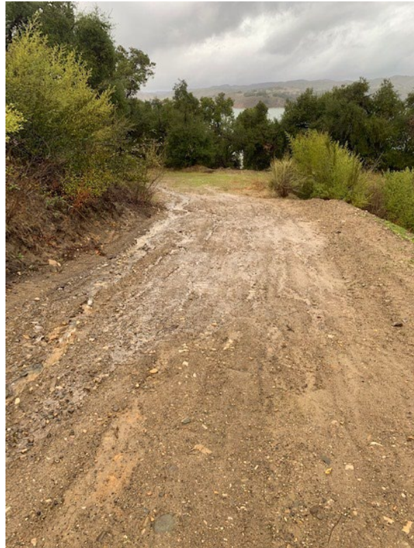
North portal access road slide repair and drainage
