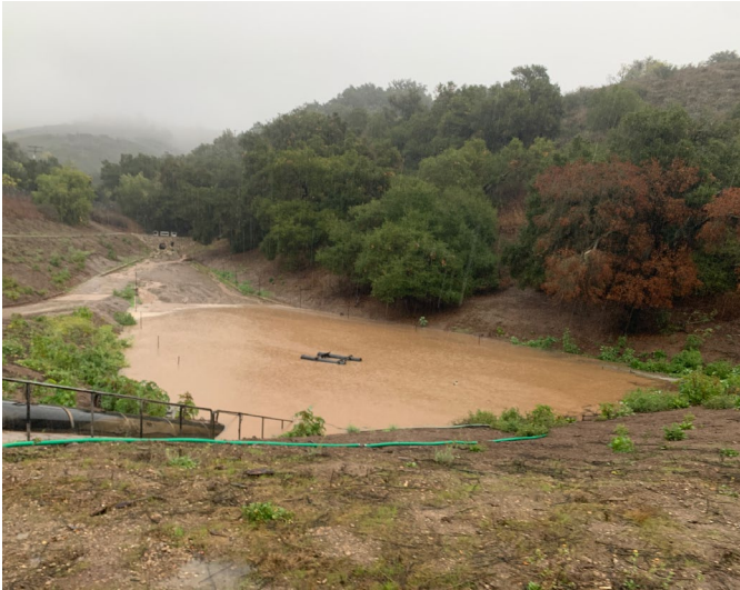
Lauro debris basin
