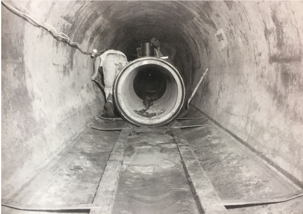
Figure 4. Historical Photo of Sheffield Tunnel Pipeline installation
