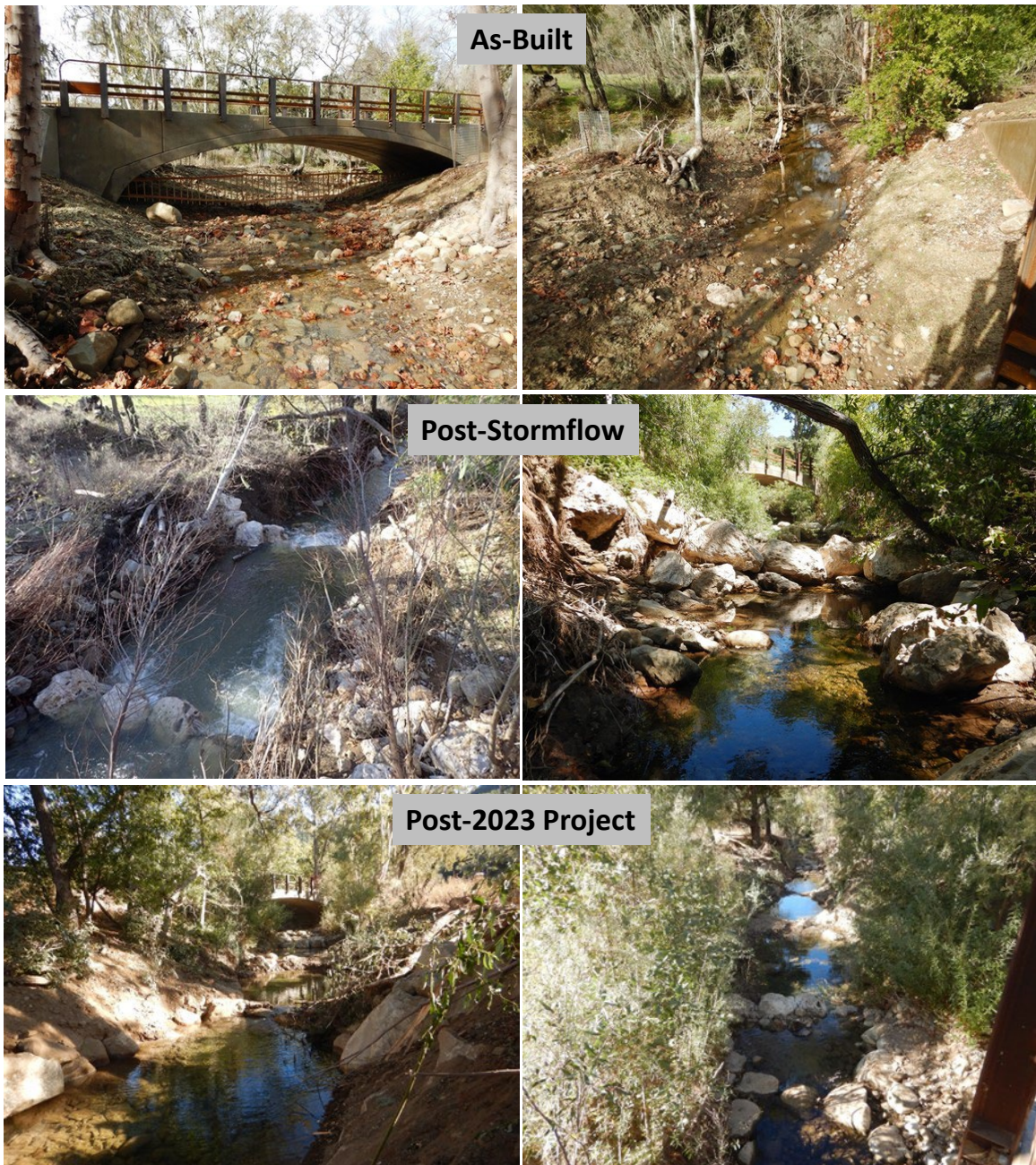
Figure 127: Quiota Creek Crossing 9 showing the As-Built, post-stormflows and post 2023 project conditions.
