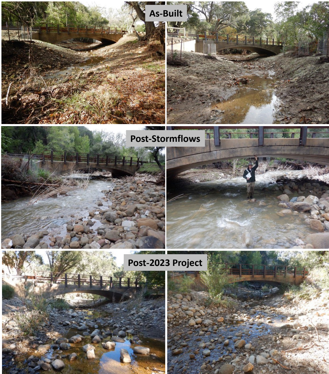
Figure 126: Quiota Creek Crossing 5 showing the As-Built, post-stormflows and post 2023 project conditions.
