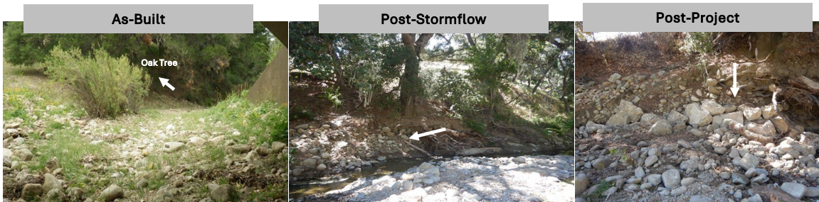
Figure 132: Quiota Creek Project at Crossing 1 showing the As-Built, post-stormflows, and post 2024 project.
