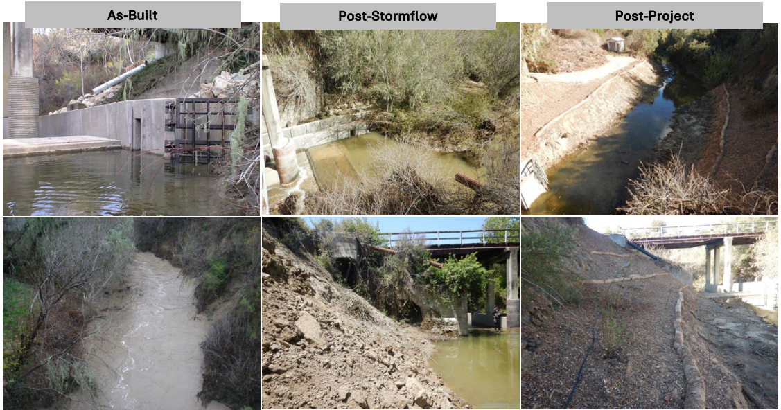
Figure 133: El Jaro Creek at Rancho San Julian Project showing the As-Built, post-stormflows and post 2023 project.
