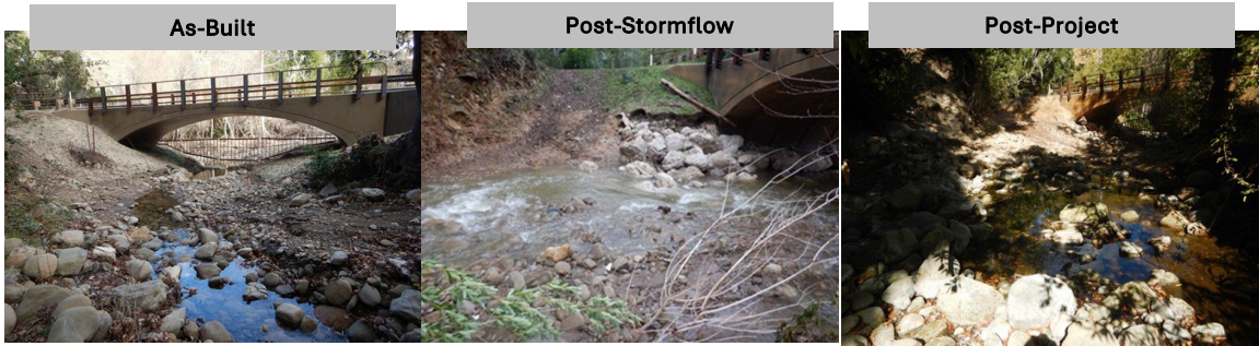
Figure 129: Quiota Creek Project at Crossing 8 showing the As-Built, post-stormflows and post 2024 project.
