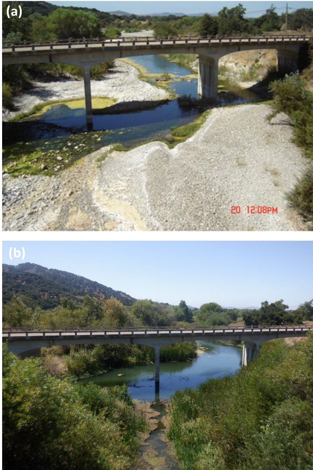
Figure 58: Photo points (M-6) collected at Highway 154 Bridge looking downstream in (a) September 2005 and (b) September 2024.
