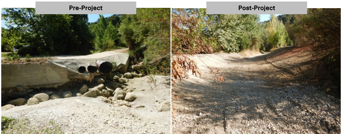
Figure 134: Quiota Creek Crossing 0B, the landowner finally removed their low flow concrete crossing that was a partial barrier to fish passage.
