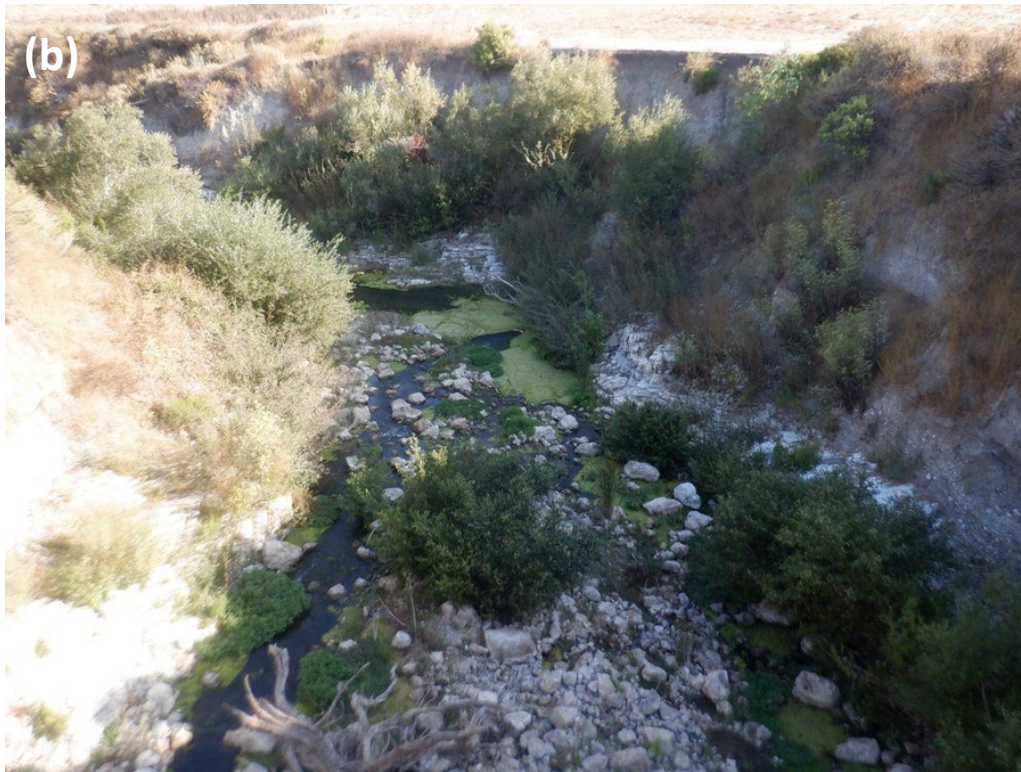
Figure 67: Photo point (T-39) collected at Salsipuedes Creek at Hwy 1 Bridge in May 2005 and (b) September 2024 (Post CalTrans Hwy 1 Bridge Replacement Project-continues to unravel).
