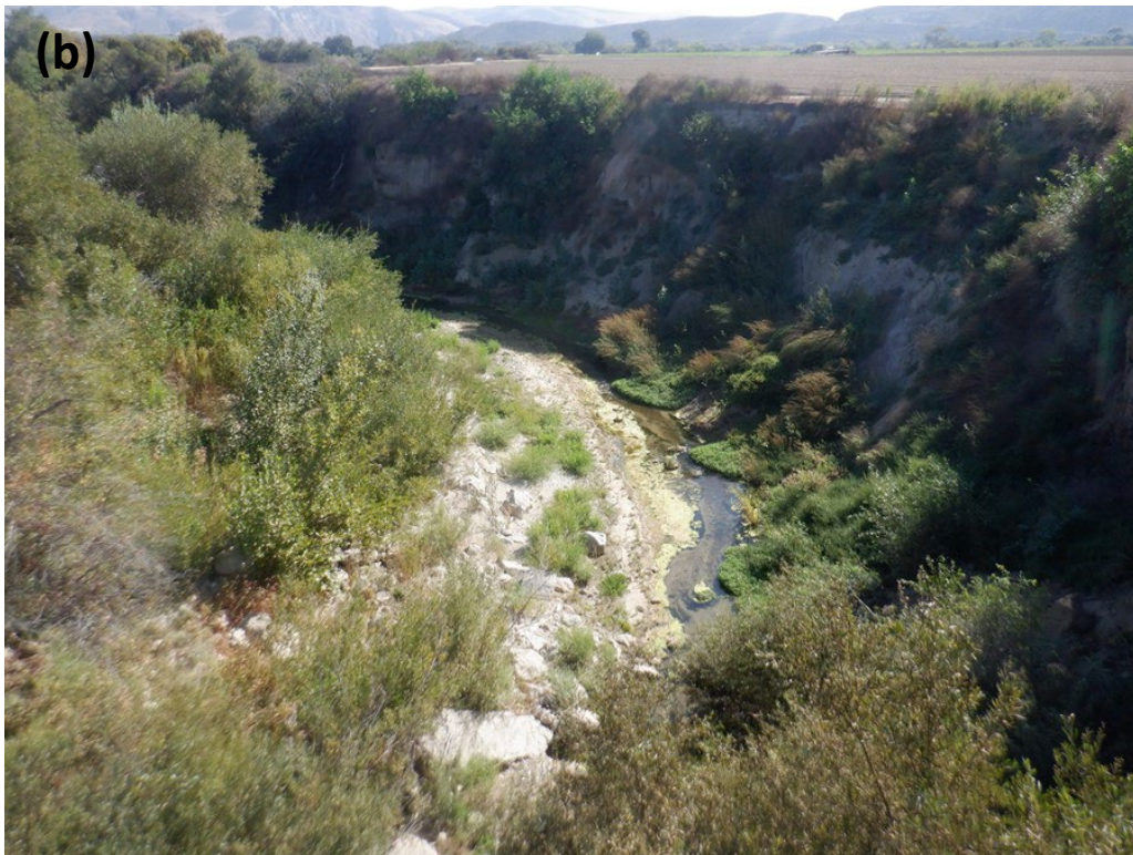
Figure 66: Photo point (T-28) collected at Salsipuedes Creek at Santa Rosa Bridge looking downstream in (a) May 2005 and (b) September 2024.
